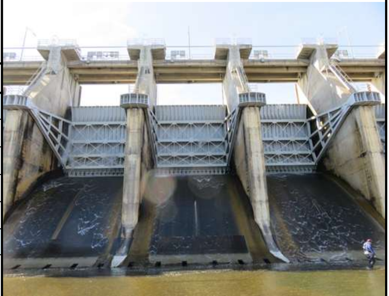
Pictured above: Downstream sides of 3 Tainter Gates at De Cordova Bend Dam.
