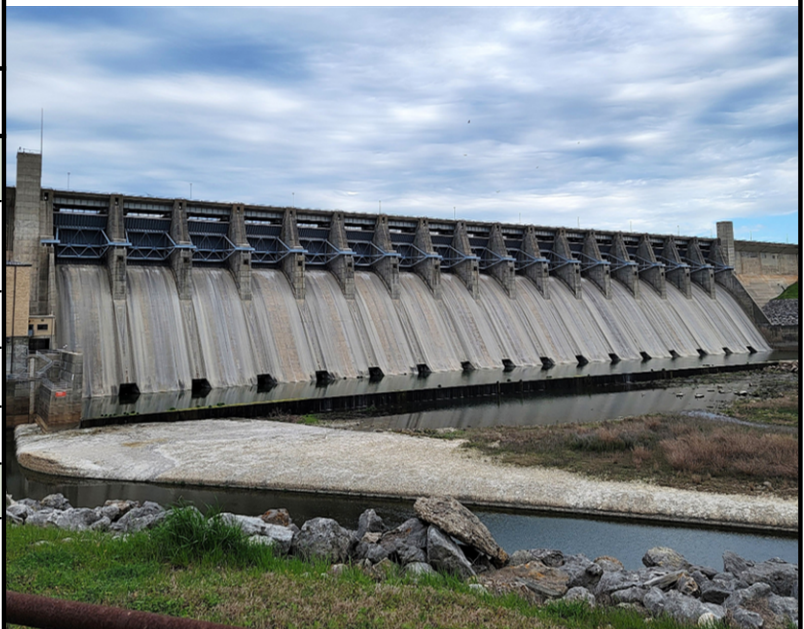
Pictured above: Lake Whitney Dam
