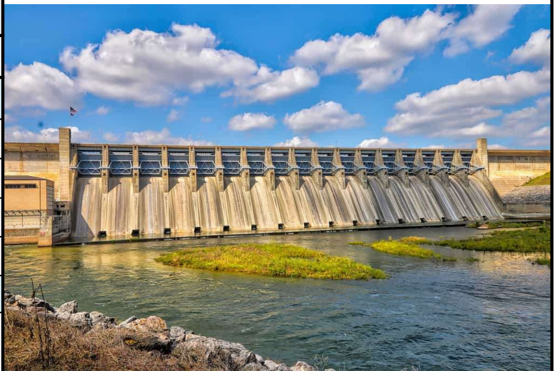
Pictured above: Lake Whitney Dam
