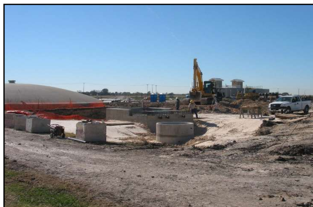
East Williamson County Plant Expansion
