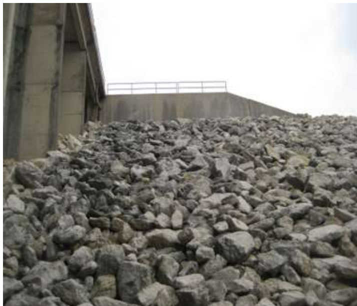
Pictured above: North, downstream embankment retaining wall
